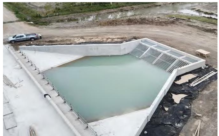
Typical Drainage Siphon Crossing
