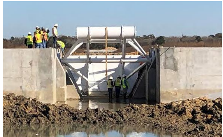
Largest Water Control Gate in Texas being installed.
