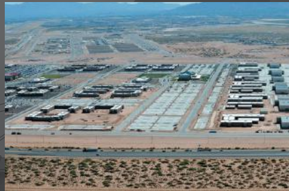
FORT BLISS EXPANSION PROGRAM ■ El Paso, Texas
