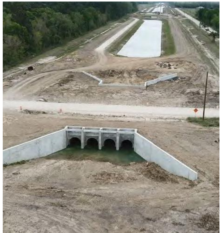
Roadway Siphon Crossing
